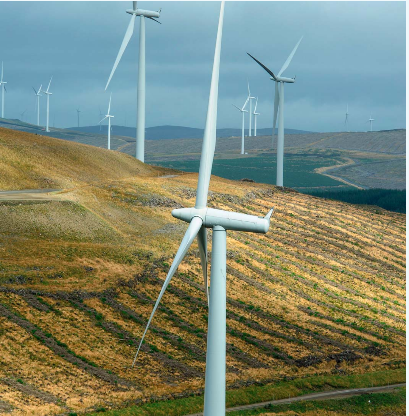
Owned partly by SSE, a portfolio company, the Clyde Wind Farm in South Lanarkshire has 206 turbines with an installed capacity 522MW generating sufficient renewable energy to power over 290,000 homes.
